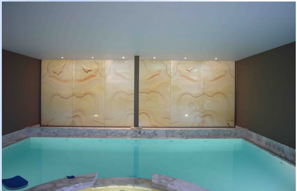
... of six STONE-GLASS panels of mm 2700x1200 in onyx (thickness mm 4) and extra-clear glasses (thickness mm 10+10)
